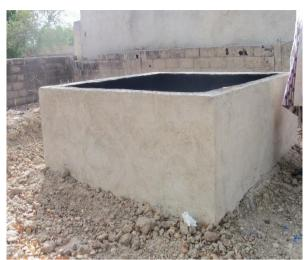
Figure 7: A brick constructed incinerator for other solid waste
